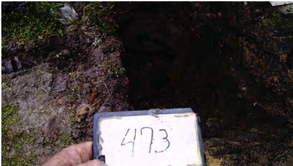
Picture 2: UST 473Dogwood tank pit.
