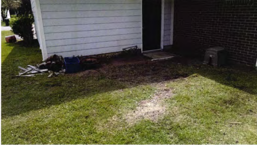
Picture 3: Site at completion of work.
